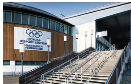
Olympia Ice Sports Stadium in Garmisch-Partenkirchen (Germany)
