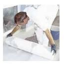
Full-surface fleece-reinforced for premium waterproofing especially above occupied rooms.
