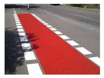
**Preco Cryl Roller-Applied Plastic 2K** is used as a textured and non-slip coating for surfaces and cycle paths, including those which run alongside the main flow of traffic. The completely elastic and non-slip surface cures in less than twenty minutes.
